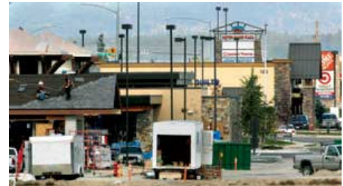
Caption: Construction workers shingle the roof of the Flathead Bank drive-through at Hutton Ranch Plaza in October of 2007. - File photo by Lido Vizzutti/Flathead Beacon
